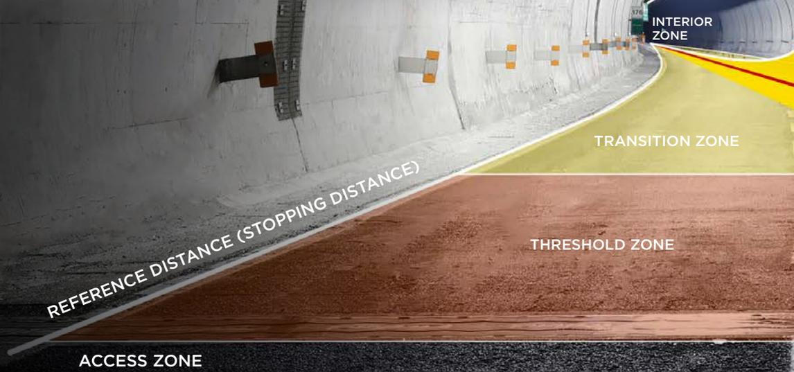
The lighting system must ensure adequate traffic safety conditions if it illuminates the tunnel in such a way as to ensure that any obstacles on the road surface are visible from a distance sufficient to allow the driver to stop the vehicle without any direct consequence or others. This condition must be ensured by the zone of "entry" to the zone of "exit" of the tunnel.
