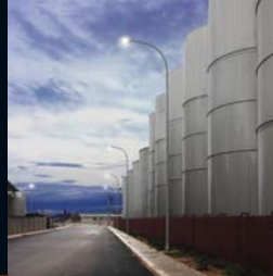
TRINITAPOLI INDUSTRIAL AREA Italy
