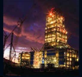
KONIAMBO NICKEL PLANT New Caledonia Australia
