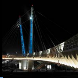
SHA LU OVERPASS Taiwan
